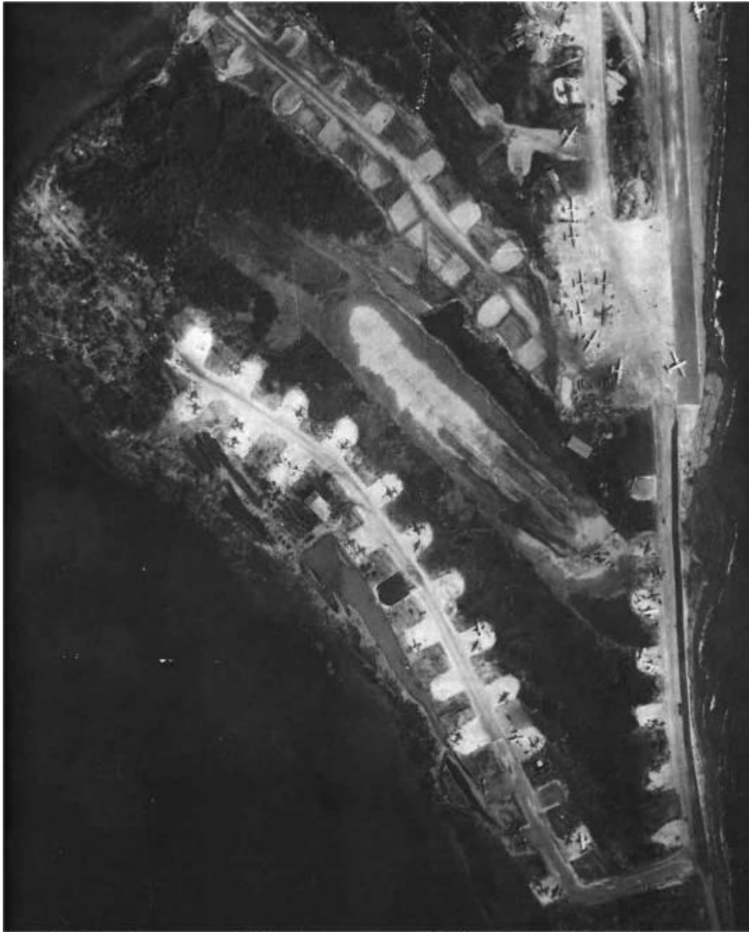
The Air Apaches were consolidating their operations at Tacloban Airstrip which was built on a peninsula jutting into the sea on the east side of Leyte Island. The hardstands at left are full of B-25s from the 345th.
